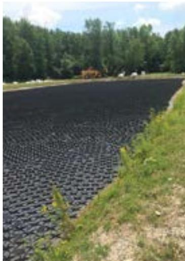
Installed in less than 4 hours, bags of discs were emptied into the basin and the cover immediately began serving as a bird deterrent, eliminating odors and keeping wildlife from coming in contact with potentially harmful de-icing fluids.
