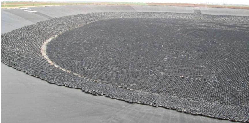
The water level in the reservoir changes 1-2 meter per day. The Hexa-Cover® Floating Cover automatically adapts to these changes.
