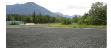
"Familiar with the Hexa-Cover<sup>®</sup>, I felt the product could nicely cover the lagoon, controlling the algae growth as the sunlight would not be able to penetrate into the water. Additionally, the Hexa-Cover<sup>®</sup> would enable the aeration process and fluctuating water levels to continue"
