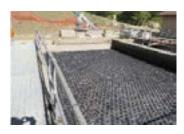
A solid cover presented safety issues, the discs did not. Summit Engineers was going to put aeration in these basins but saw a sample of the Hexa-Cover<sup>®</sup> product, called references then recommended the Hexa-Cover<sup>®</sup> installation. It penciled out better than aeration. That was important to this design build project, which Western Water Constructors, Inc. did with Summit.
